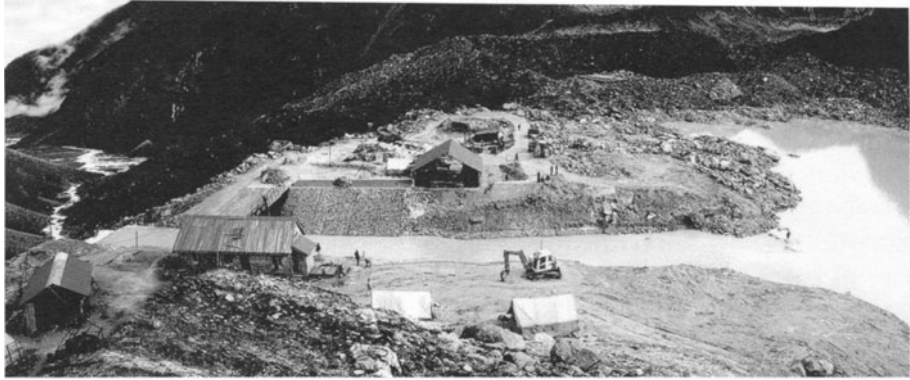
Figure 3: The nearly completed spillway at Tsho Rolpa (4,500 m), Rolwaling Himal, Nepal, in 2000. The lake level was lowered successfully by 3.5 m following construction of the new spillway and sluice gates. It took from April 1999 to July 2000 to complete the works at a cost of ca $3 million. Heavy machinery had to be flown to the site in bits and reconstructed at site. Glacier ice is still present within the moraine dam (right-hand side of picture). Although the glacial hazard has been reduced significantly, it has been recommended that the lake level should be drawn down at least a further 11.5 m to ensure an adequate factor of safety for the 150-m high moraine dam (Photograph © Reynolds Geo-Sciences Ltd, 2000).
