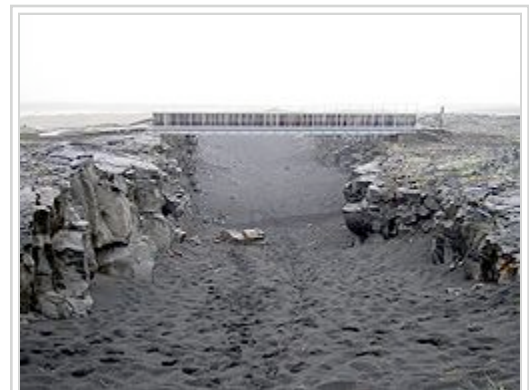
Bridge across the Álfgjá rift valley in southwest Iceland, the boundary between the Eurasian and North American continental tectonic plates.
