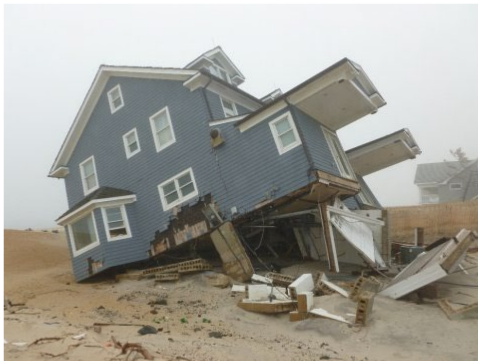
Figure 13: House in Mantoloking Knocked Off Foundation by Superstorm Sandy Storm Surge 284
